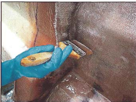
Impregnating the fibres
